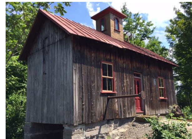
Figure 10 La centrale Dunn
